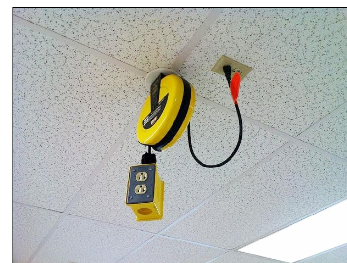
2 CEILING OUTLET EXAMPLE SCALE :: NTS
